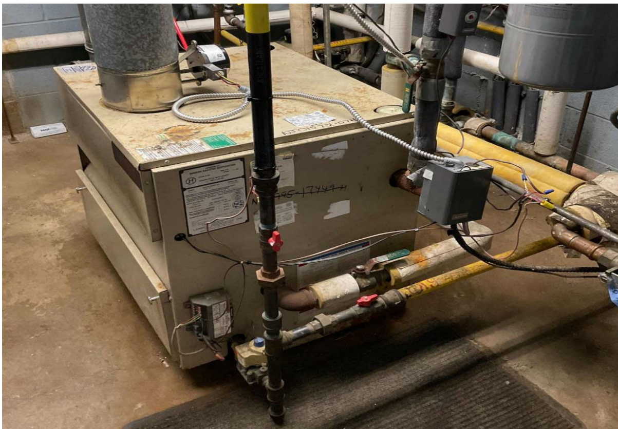
Hot Water Boiler
