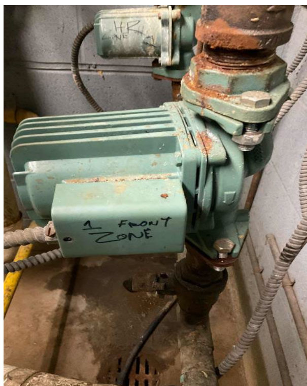
Heating Hot Water Pumps
