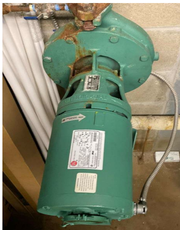
Heating Hot Water Pumps
