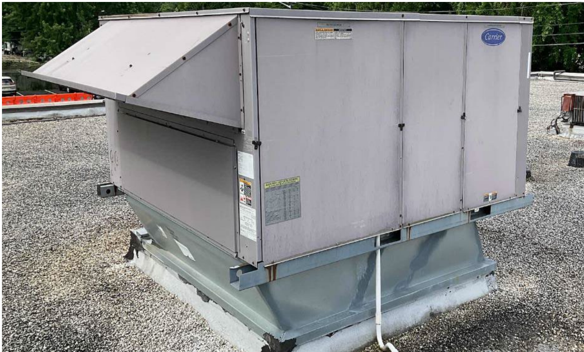
Packaged Rooftop Unit
