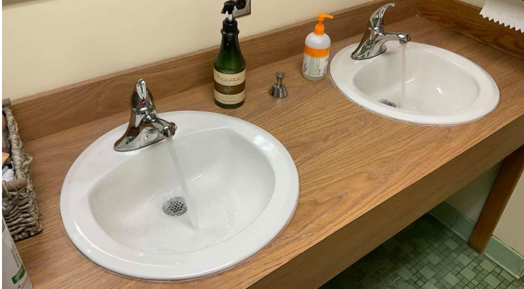
Typical Restroom Sinks
