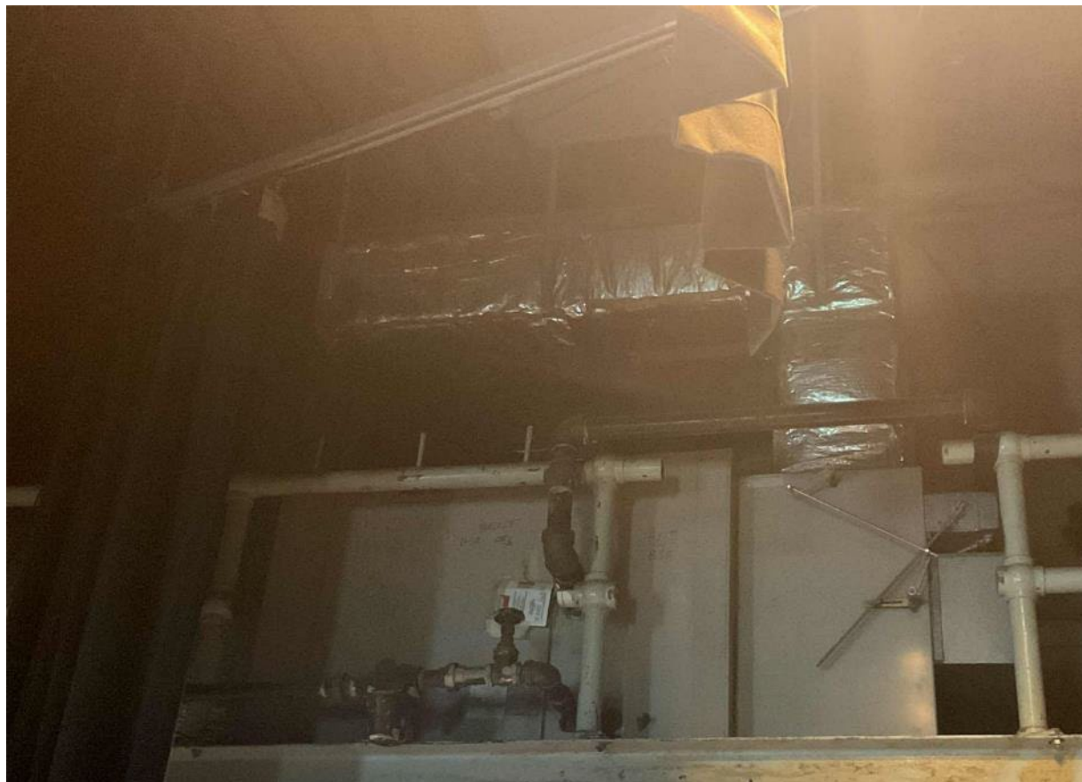
Air Handling Unit
