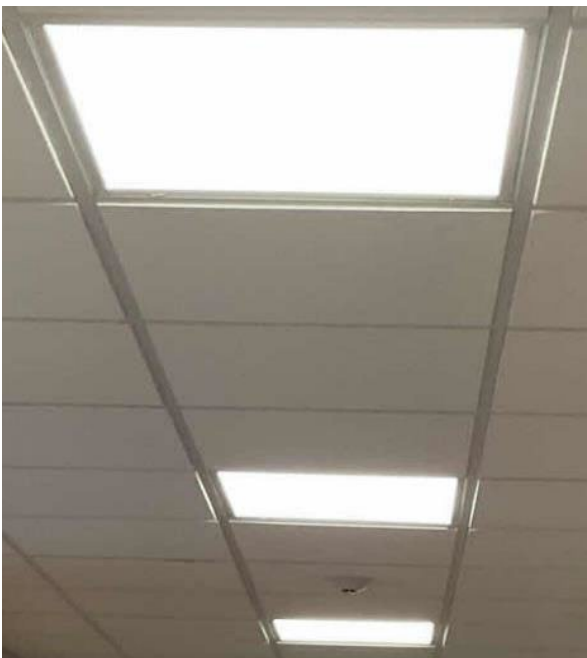
Fluorescent T8 Fixtures
