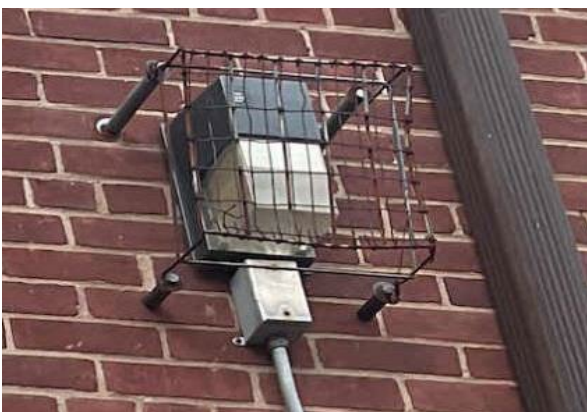
Exterior CFL Fixture
