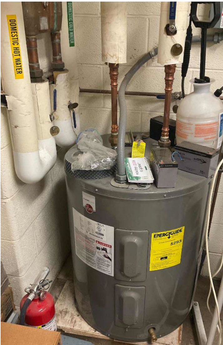
Water Heater & Circulation Pump
