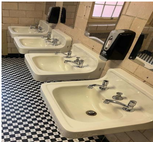
Typical Restroom Sinks
