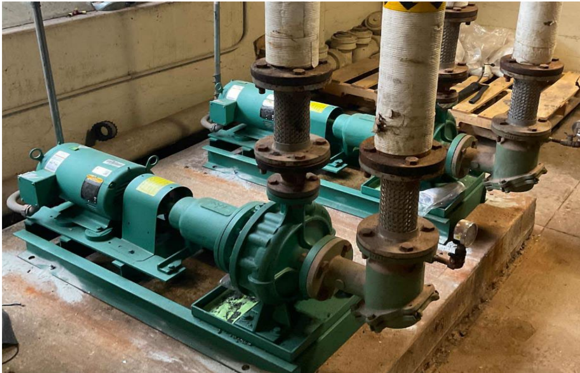
Heating Hot Water Pumps
