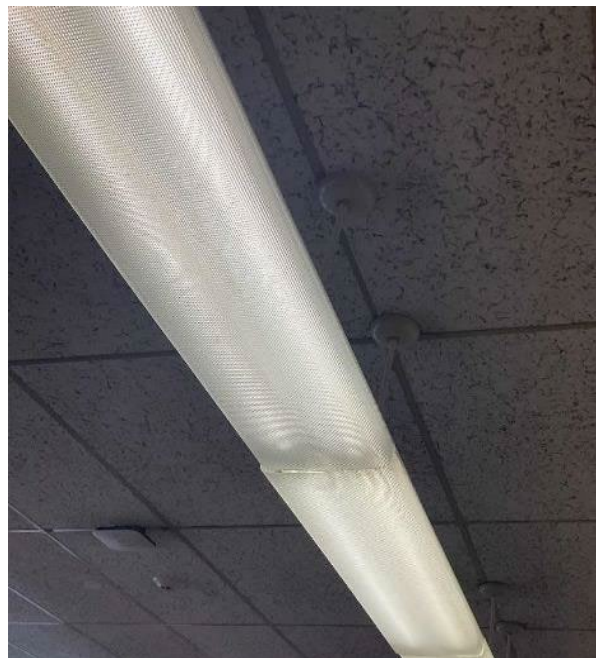
Fluorescent T8 Fixtures
