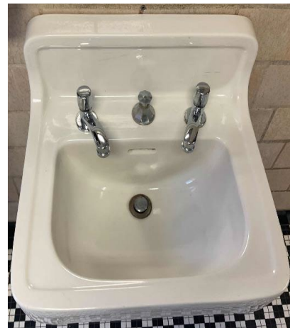
Typical Restroom Sinks
