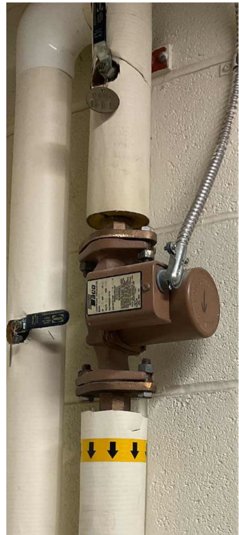
Water Heater & Circulation Pump
