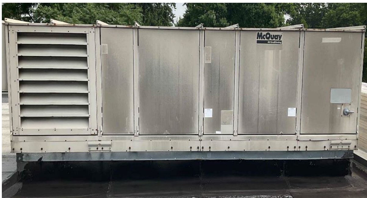
Rooftop Unit - Gymnasium
