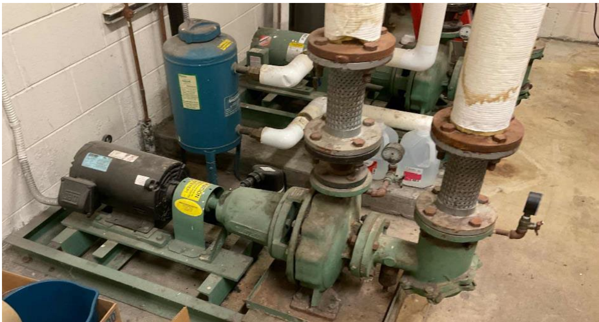
Heating Hot Water Pumps
