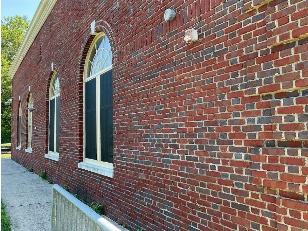
Building Walls and Windows
