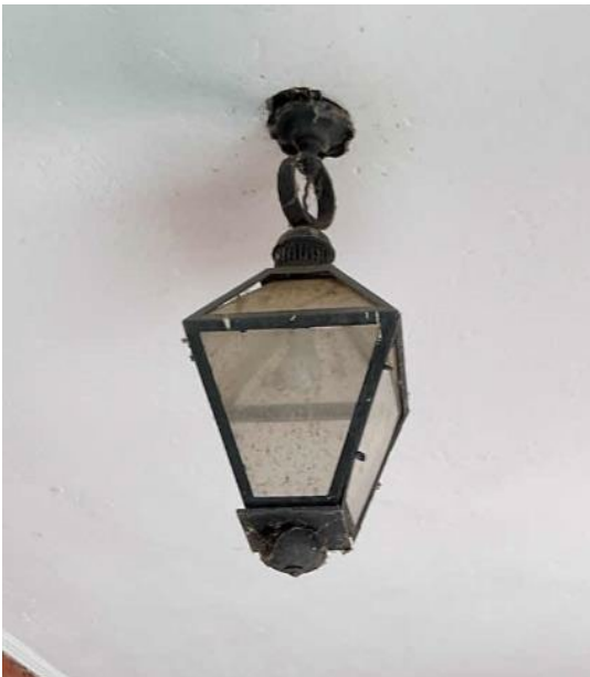
Exterior LED Fixtures
