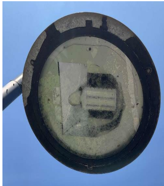
Exterior LED Fixtures
