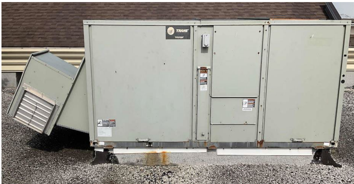
Rooftop Unit – Library
