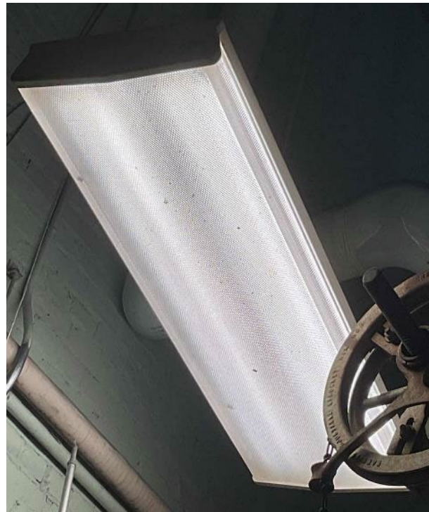
Fluorescent T8 Fixtures
