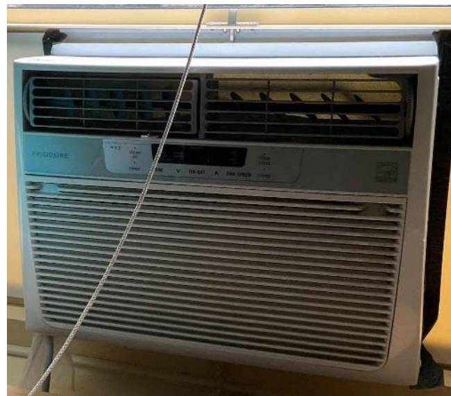
Window AC Unit
