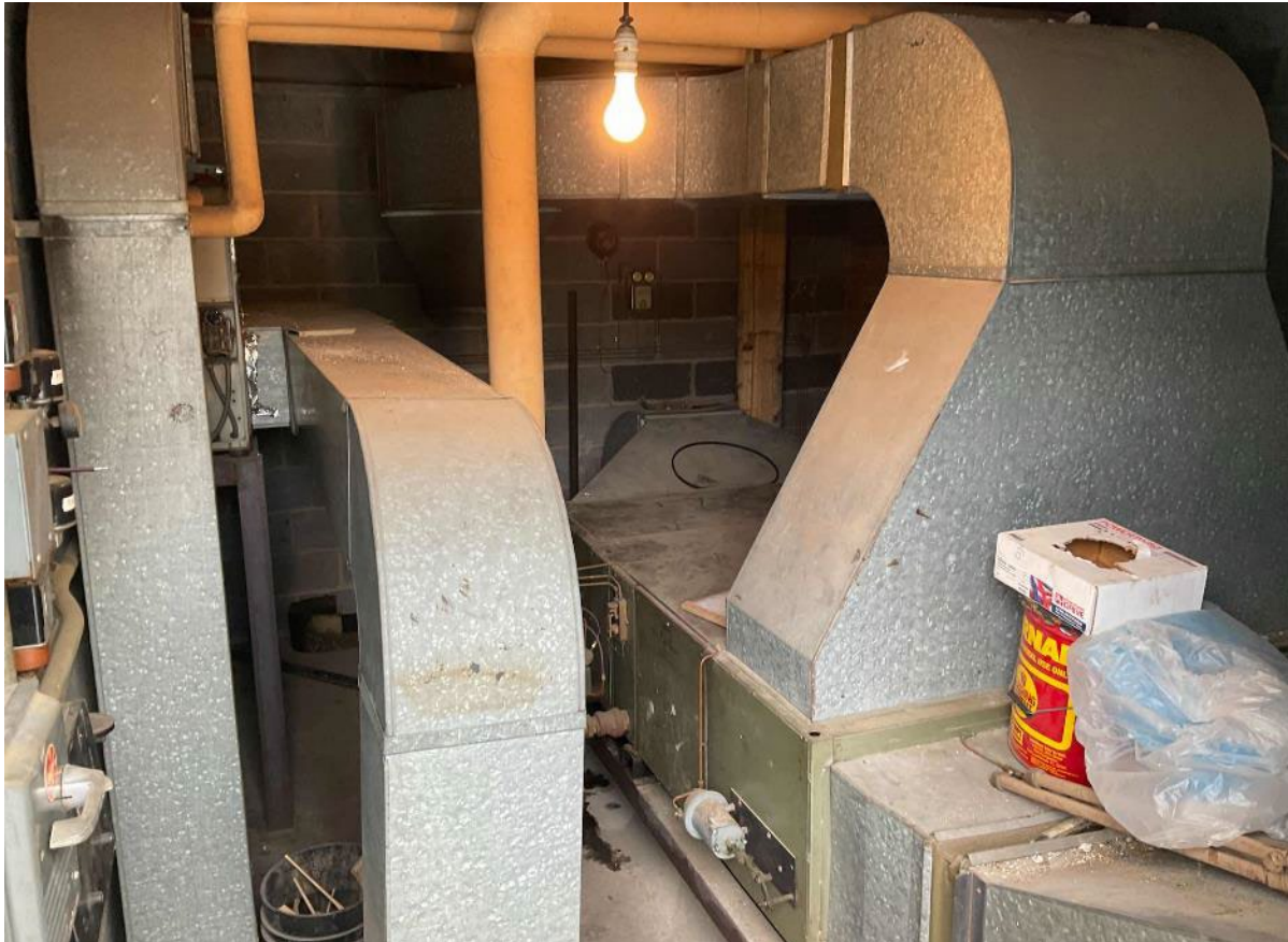
Air Handling Unit
