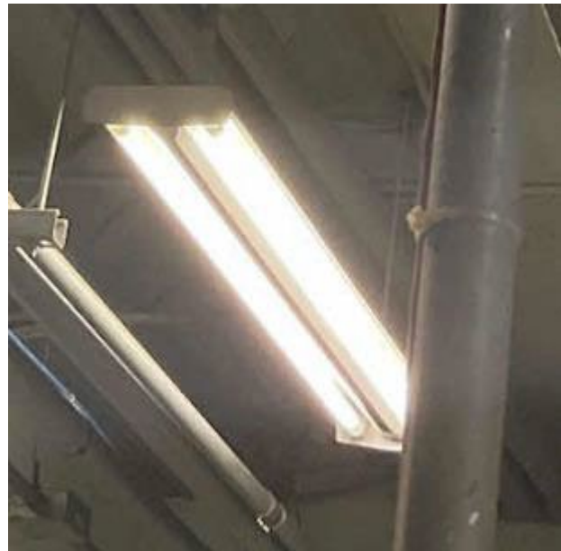
Fluorescent T8 Fixtures
