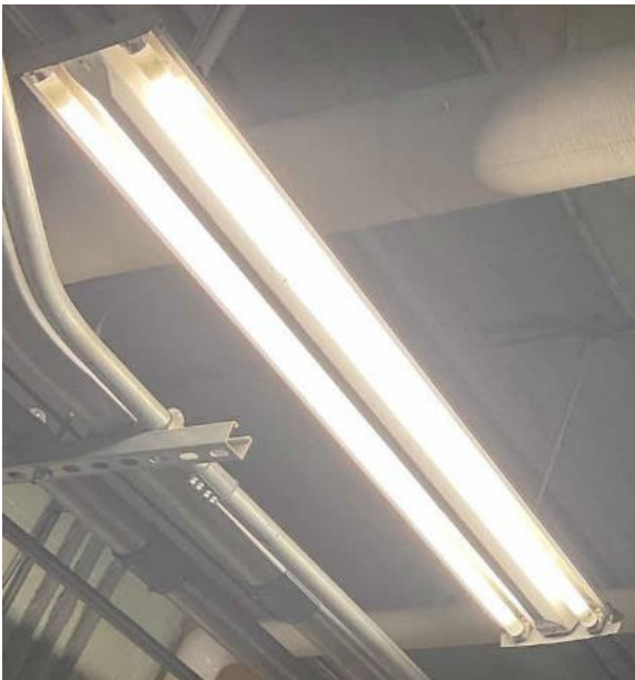
Fluorescent T8 Fixtures
