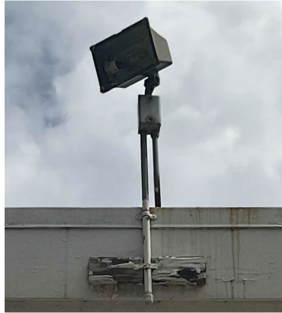
Exterior MH Fixture
