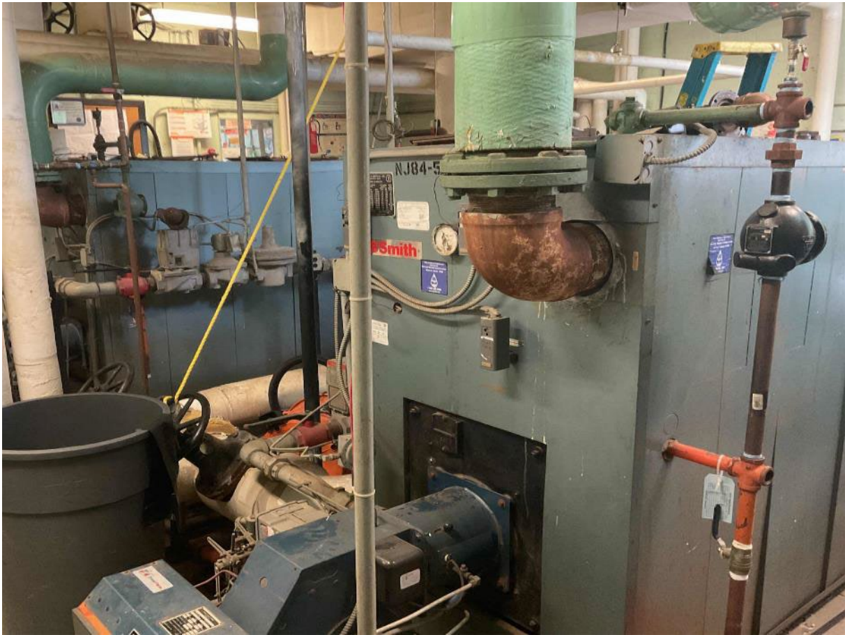
Hot Water Boilers
