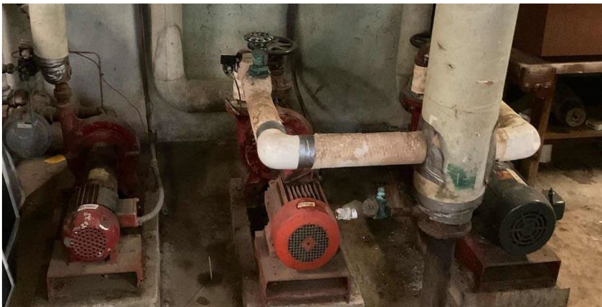
Heating Hot Water Pumps
