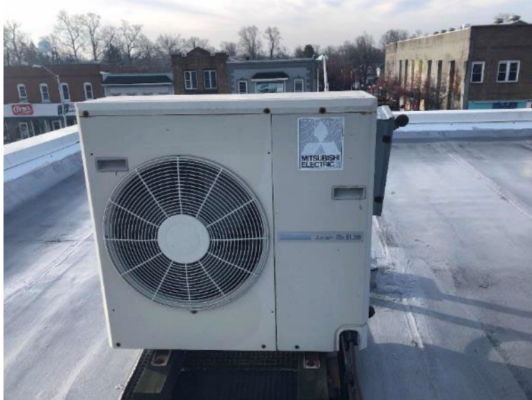
Outdoor Condensing Unit
