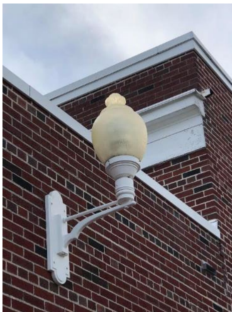
Exterior Fixture with LED Bulb
