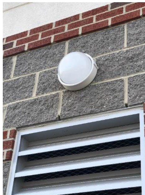
Exterior Fixture with Incandescent Bulb
