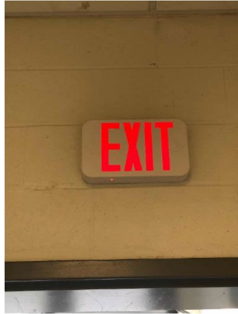
LED Exit Sign
