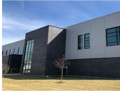
Side of Building
