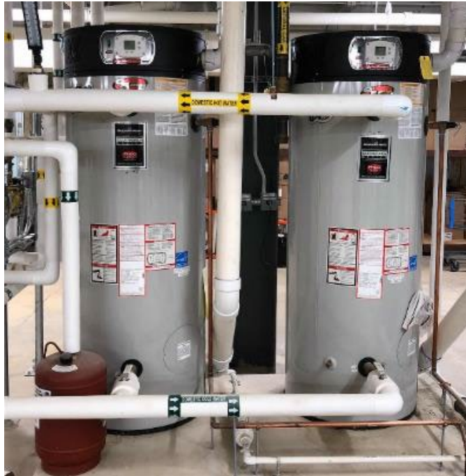
Storage Hot Water Tanks
