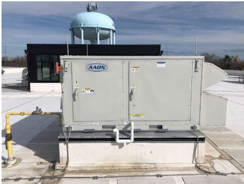
Packaged Rooftop Unit
