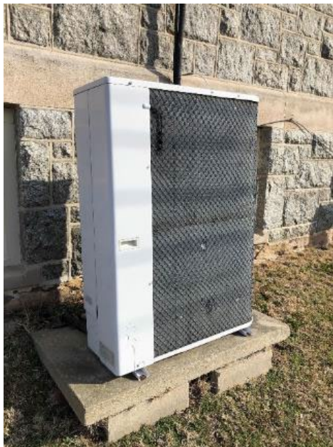
Outdoor Condensing Unit
