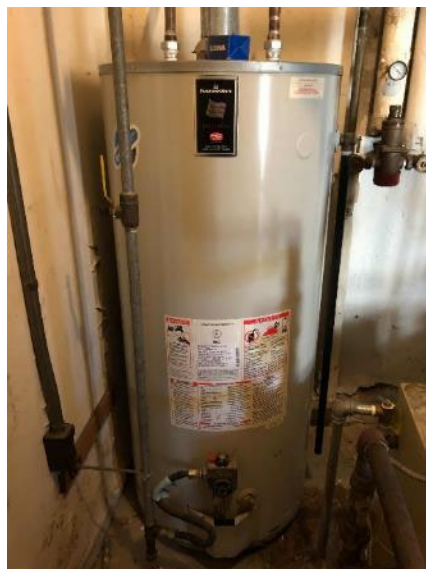
Storage Water Heater
