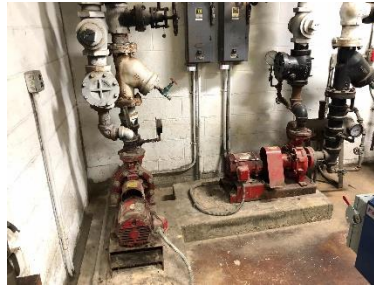
Heating Hot Water Pumps
