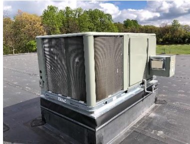
Packaged Roof Top Units (RTUs)
