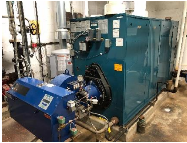
Hot Water Boiler
