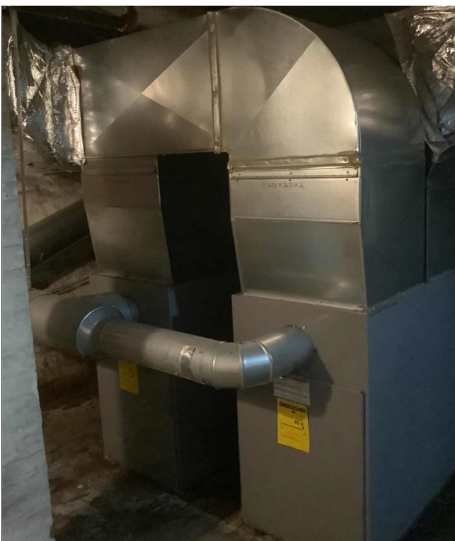
118 MBh Output Furnace Unit
