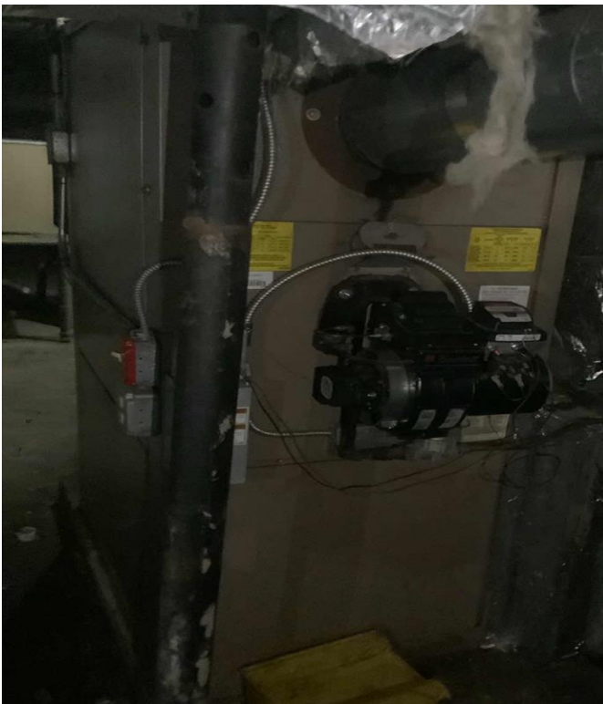
284 MBh Output Furnace Unit
