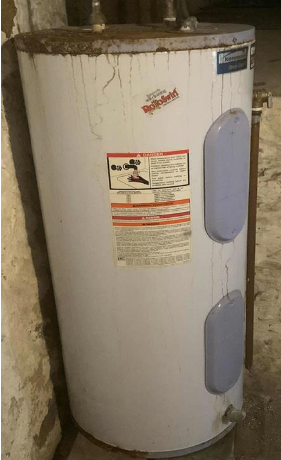
Electric Storage Tank Water Heater
