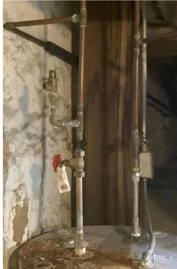
Electric Storage Tank Water Heater
