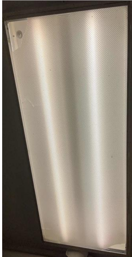
Linear Fluorescent T12 and T8 Fixtures
