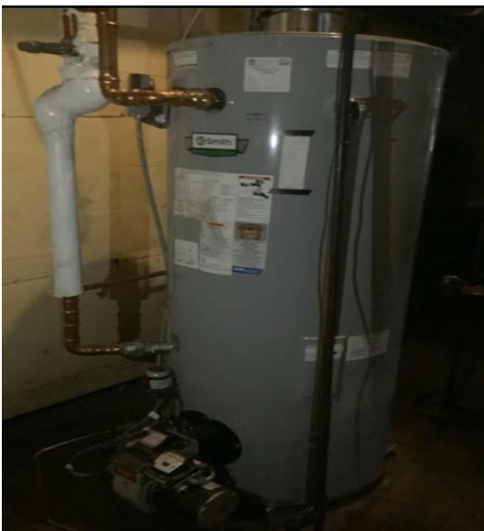
Oil-Fired Storage Tank Water Heater
