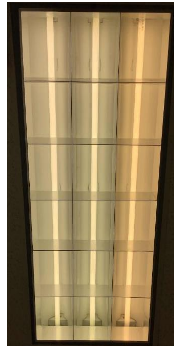
4-Foot T8 Linear Fluorescent Lamps
