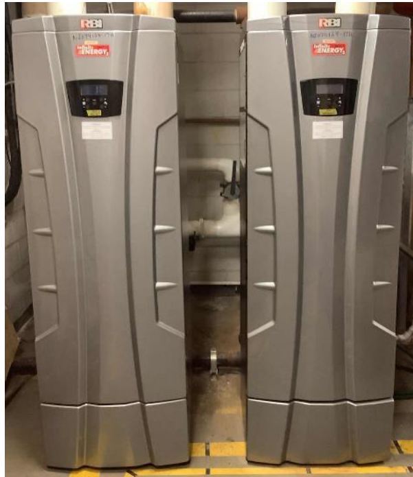
Condensing Hot Water Boilers
