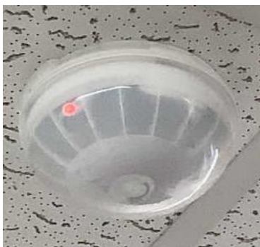
Ceiling Mounted Occupancy Sensor
