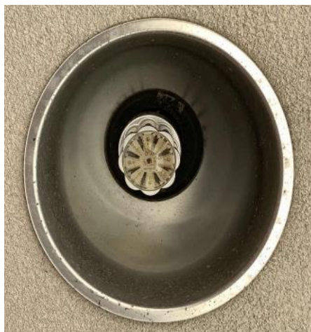
Recessed Can LED "Corn" Bulb
