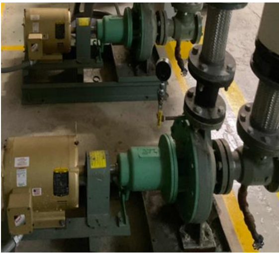
10 hp Variable Flow Hot Water Pumps
