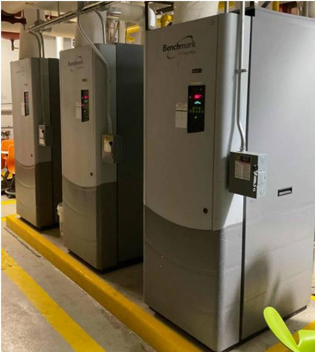
Condensing Boilers
