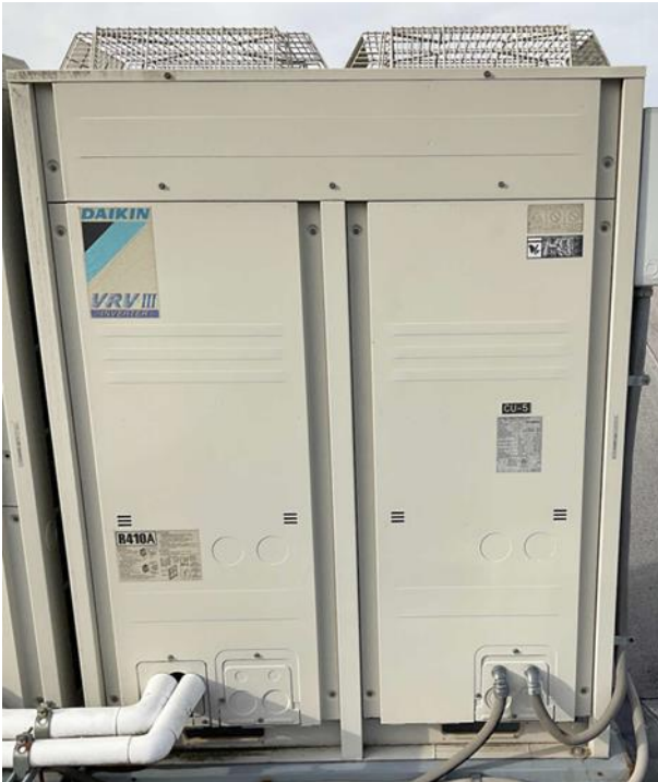
Typical Daikin VRV Heat Pump - CU-6
