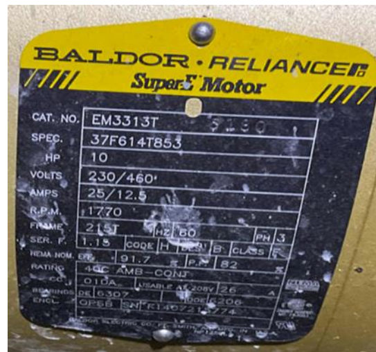
10 hp Variable Flow Hot Water Pumps
