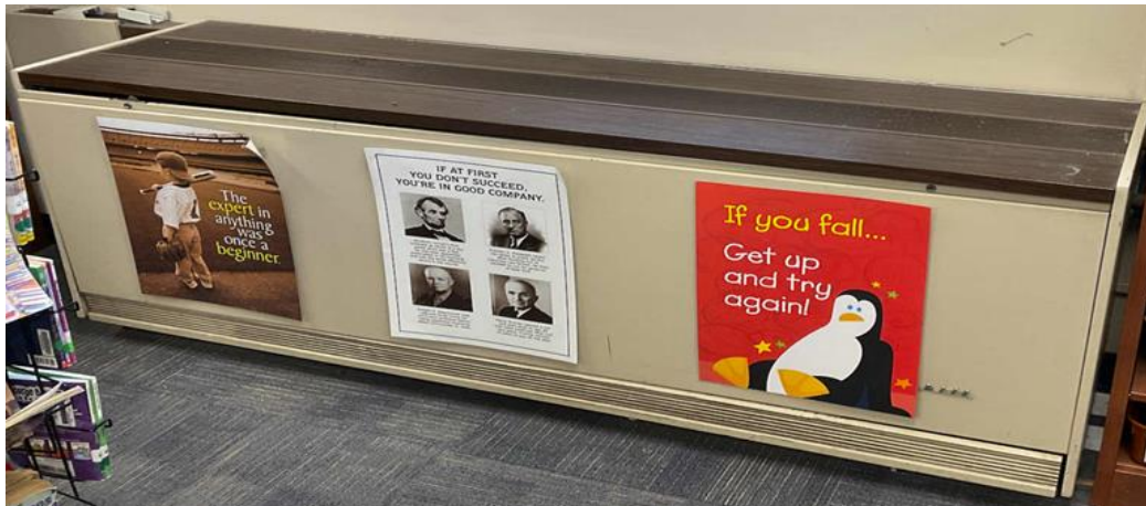
Typical Unit Ventilator
