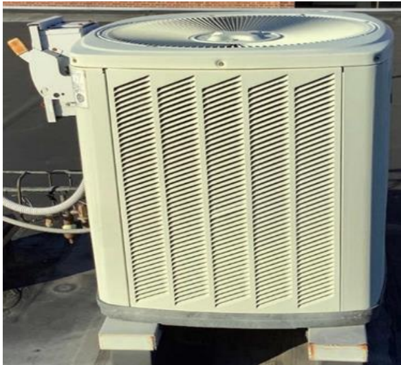
Typical Trane Condensing Unit
