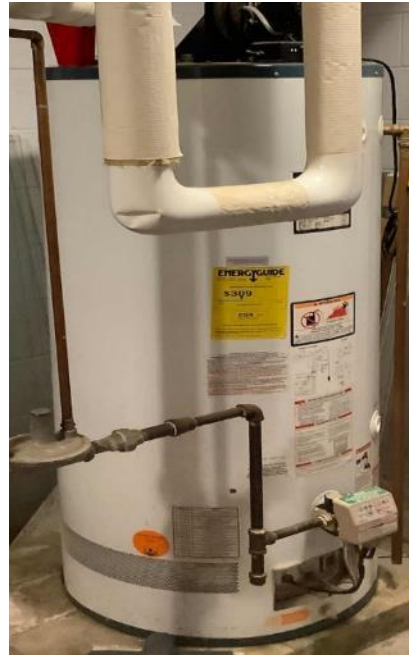
Gas Fired Domestic Hot Water Heater
