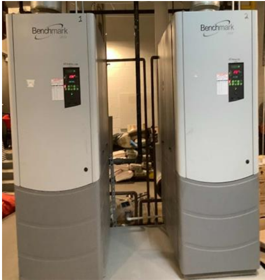
Condensing Boilers - Addition Building
