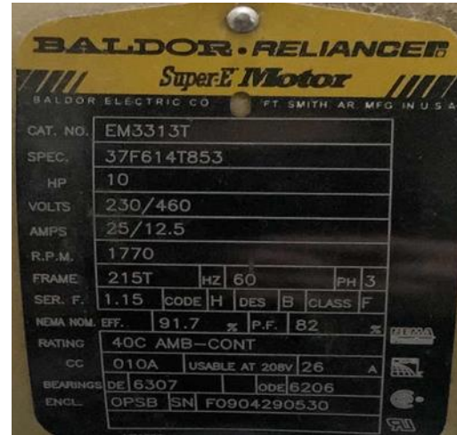
10 hp Hot Water Pumps - Original Building
