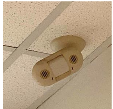
Ceiling Mounted Motion Sensor
