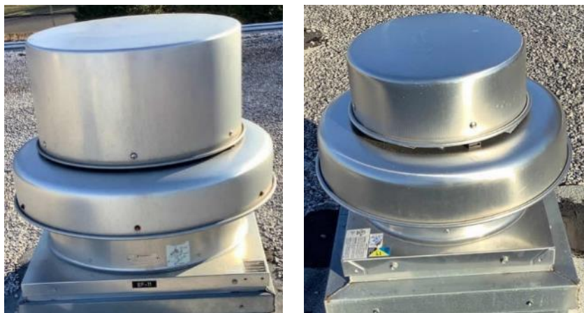
Roof Exhaust Fans
