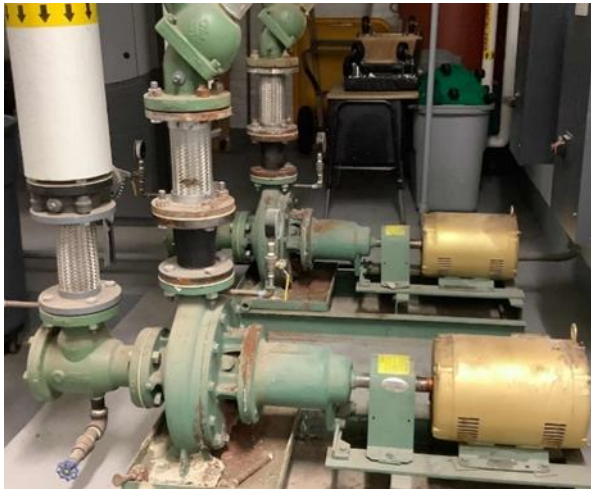
10 hp Hot Water Pumps - Original Building
