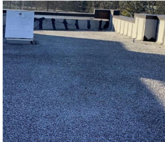
Flat Roof Section with Covering of Gravel
