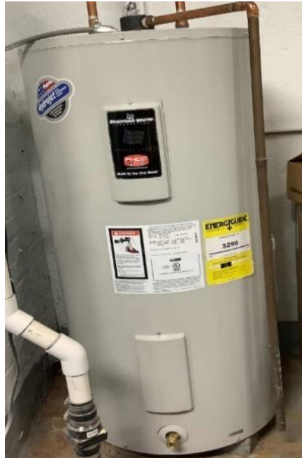
Electric Domestic Hot Water Heater
