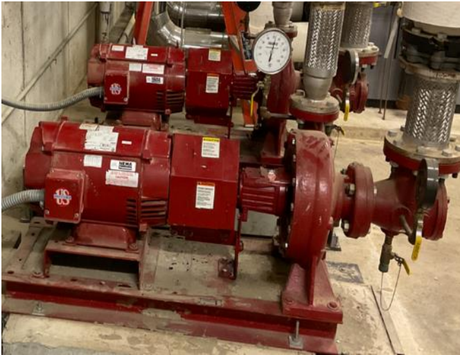
15 hp Hot Water Pumps PIP2 - Primary Center
