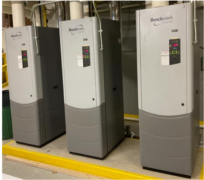
Condensing Boilers
