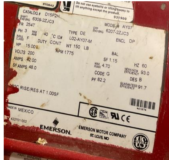
15 hp Hot Water Pumps PIP2 - Primary Center
