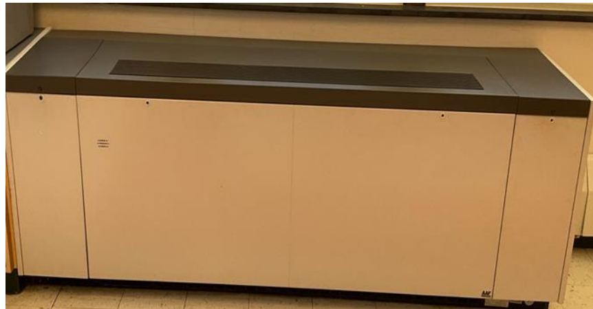
Typical Classroom Unit Ventilator
