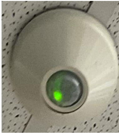
Ceiling Mounted Occupancy Sensor
