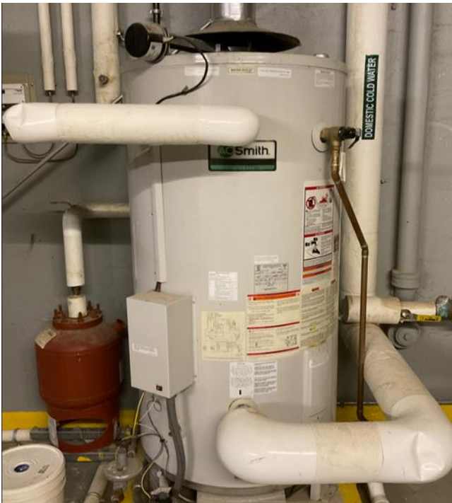
Gas-Fired Water Heater - Original Building
