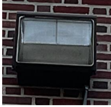
Metal Halide Fixture
