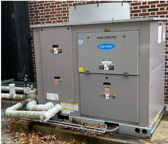
105 Tons Carrier Chiller
