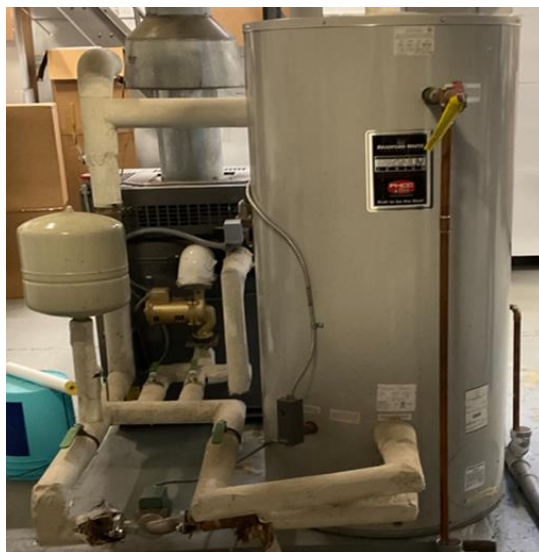
119-Gallon Separate Tank
