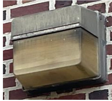
High-Pressure Sodium Fixture
