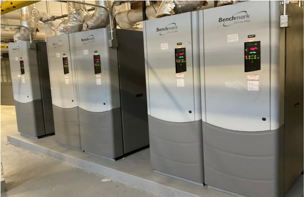
Aerco Condensing Boilers
