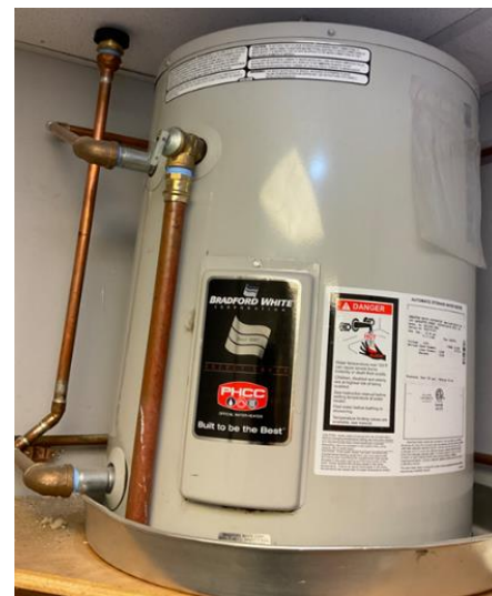
19-Gallon Electric Water Heater
