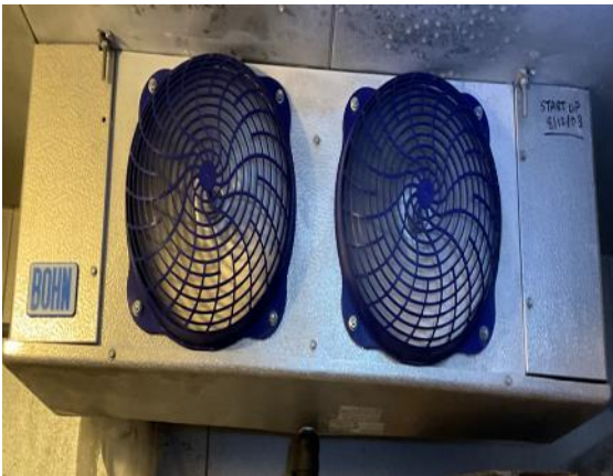
Walk-in Cooler Evaporator
