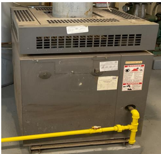
Main Domestic Hot Water Boiler
