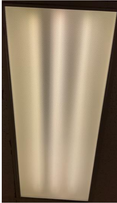
Linear Fluorescent T8 Fixtures
