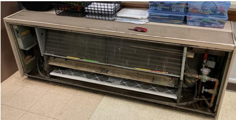
Typical Classroom Unit Ventilator
