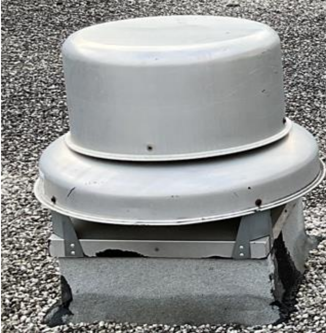
Typical Exhaust Fan
