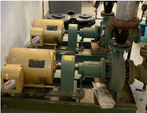
25 hp Variable Flow Pumps
