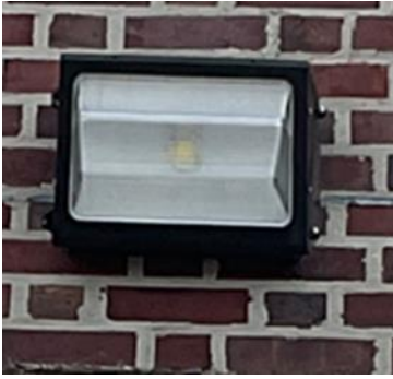
Exterior Wall Mounted LED
