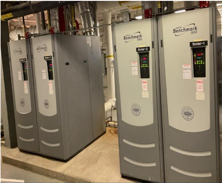
AERCO Condensing Boilers
