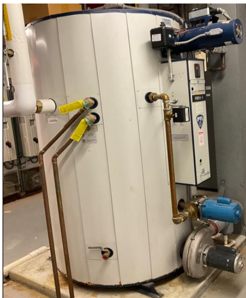
Condensing Storage Tank Water Heater
