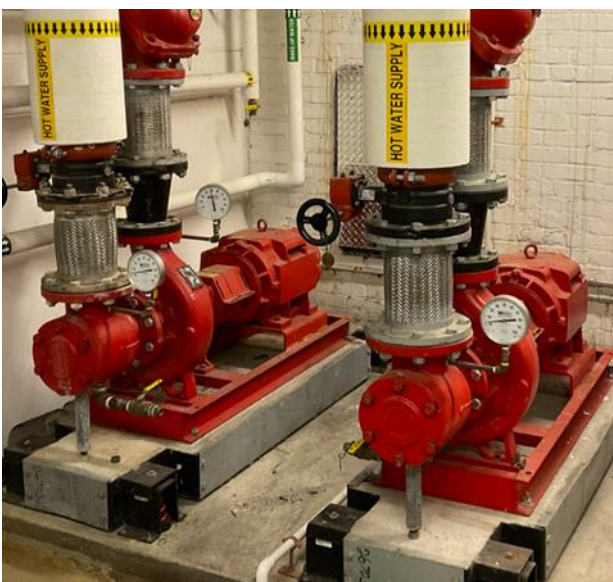
25 hp Variable Flow Pumps
