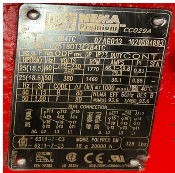
25 hp Variable Flow Pumps
