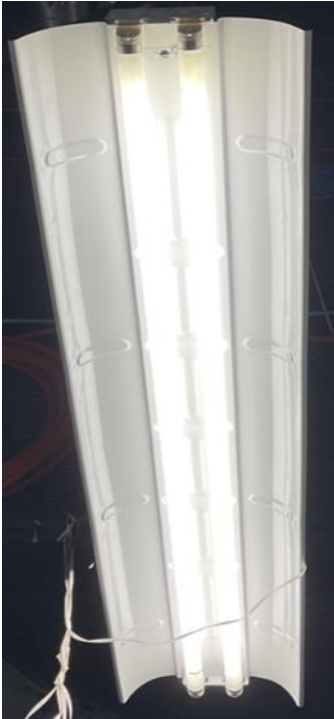
Linear Fluorescent T8 Fixture
