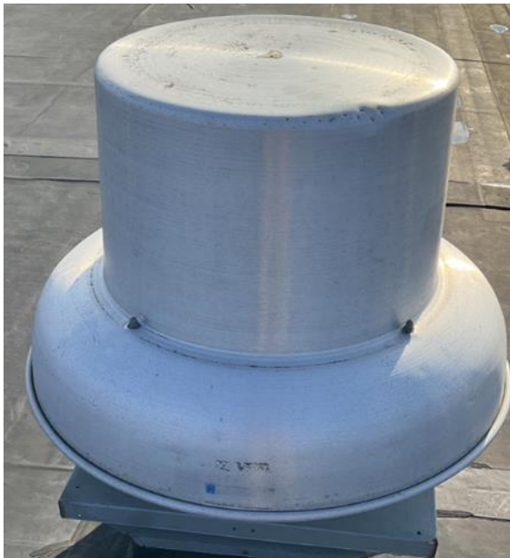
Typical Exhaust Fan
