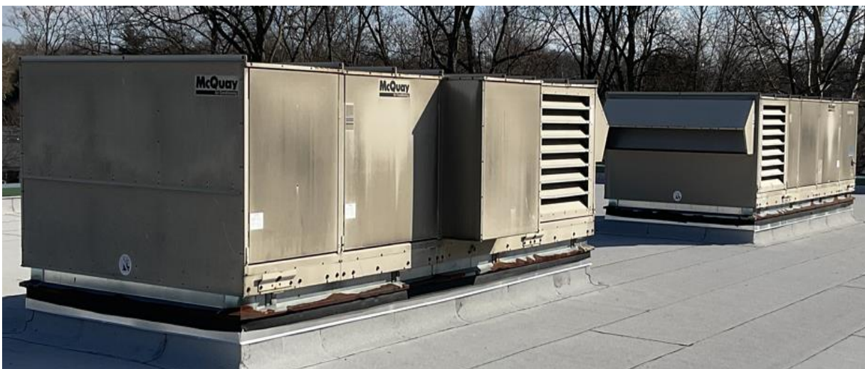
RTU-X and RTU-X2
