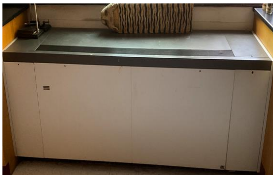
Typical Classroom Unit Ventilator
