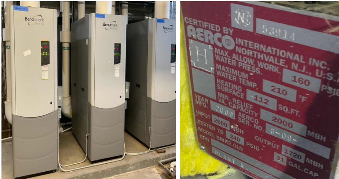
Condensing Boilers
