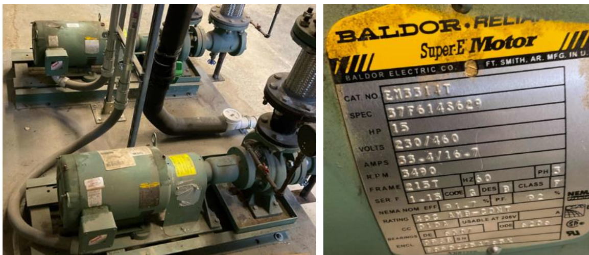
15 hp Variable Flow Pumps
