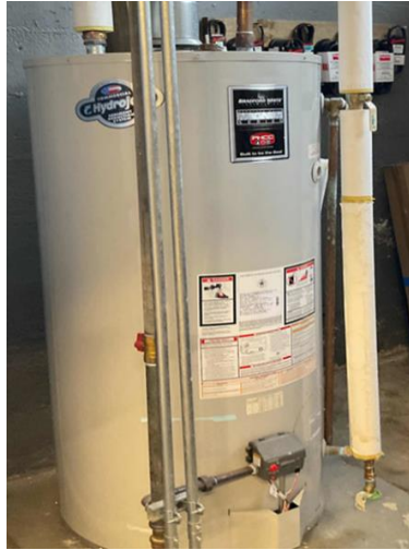
100 Gallon Gas-Fired Storage Tank Water Heater
