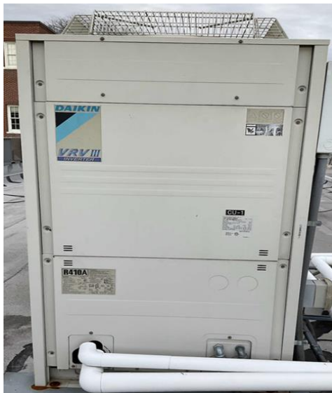
Typical Daikin VRV Heat Pump – CU-1
