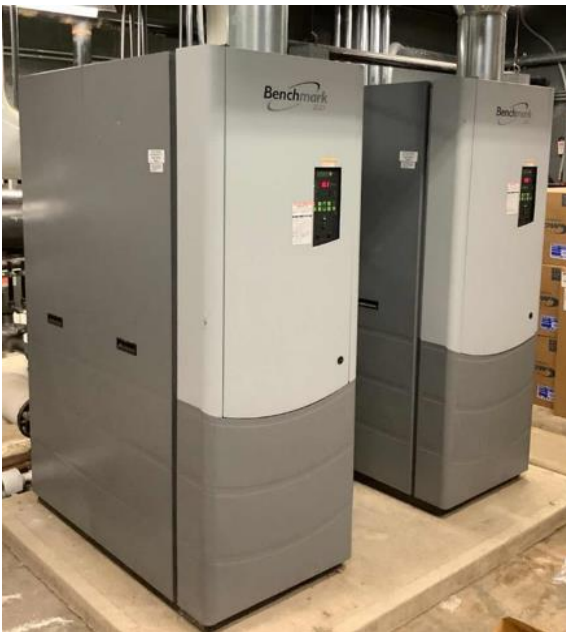
Heating Hot Water Boilers
