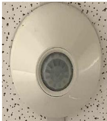
Ceiling Mounted Occupancy Sensor
