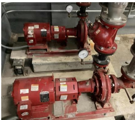
Heating Hot Water Pumps
