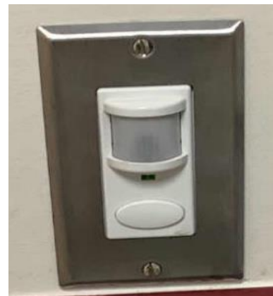
Wall Mounted Occupancy Sensor
