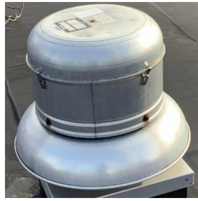
Roof Exhaust Fans
