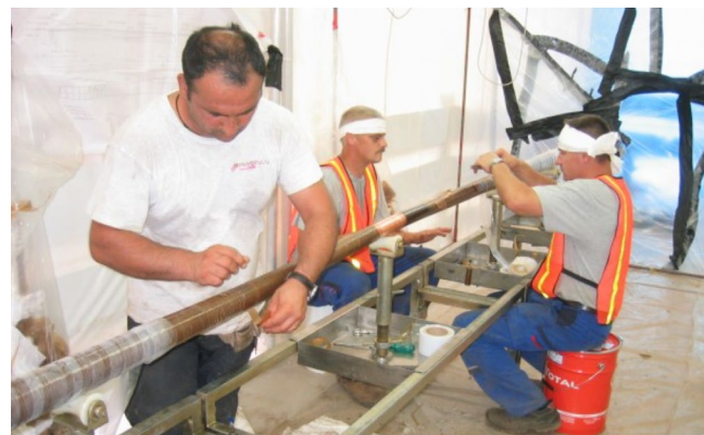
Splicing of cables along the Wantagh Parkway
